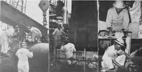
THE TURNAROUND features both big and little jobs. A derrick is used to position one of the base supports for a reaction chamber, left. The flared chamber base, center, is positioned on its new foundation. Chipping and cleaning, right, are important, too.
